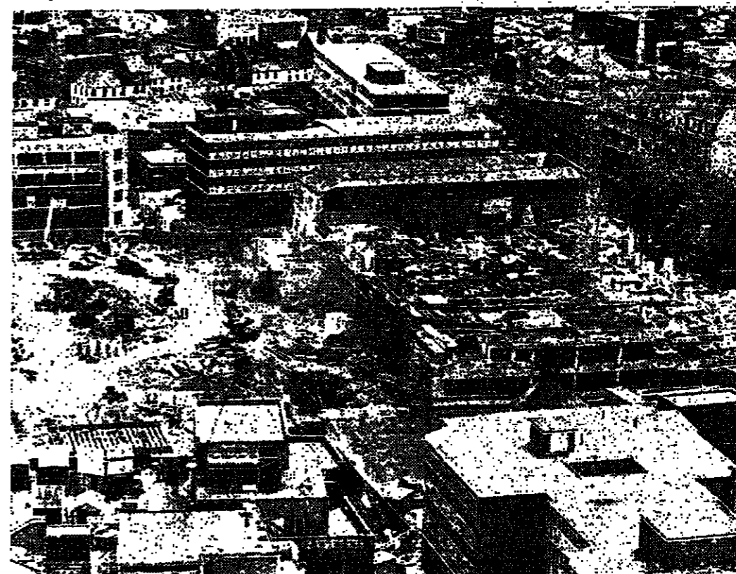
Work on Cardiff's long-delayed £50m. city centre redevelopment scheme is helping to soak up unemployment stemming from steel redundancies.
